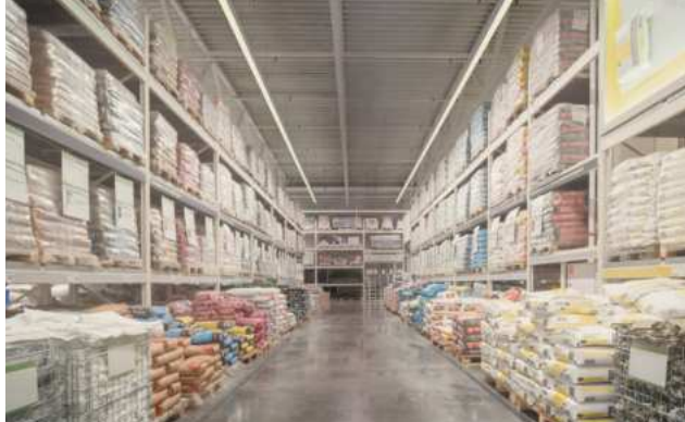
Double asymmetrical continuous light line in the DIY store 200109
