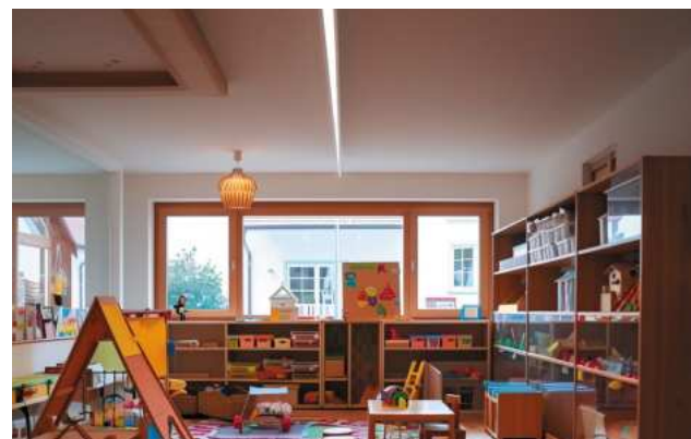
TRIAC dimmable ceiling mounted light in kindergarten 200110
